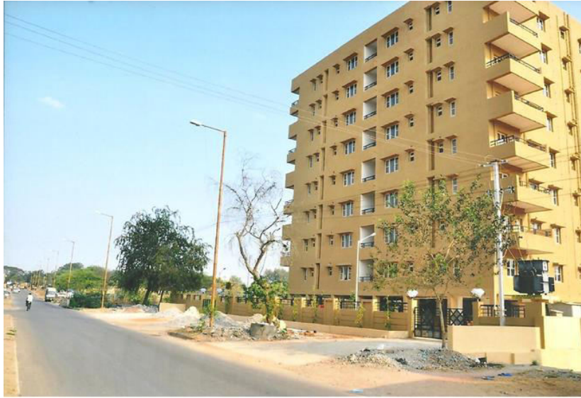
Work in progress at Lingampally Phase-III
