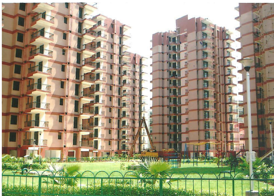
Work in progress at Sonepat
