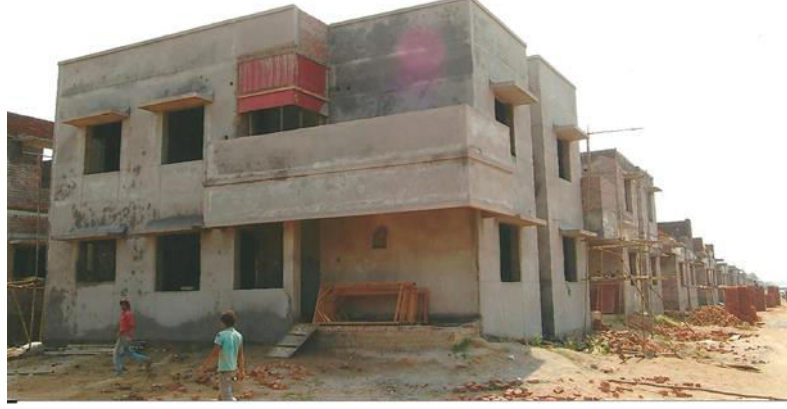
Work in progress at Chennai Phase-IIA
