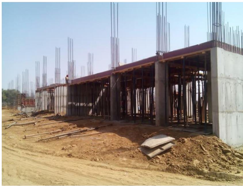
Work at Jaipur Phase-III
