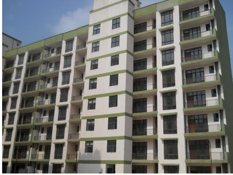
Work in progress at Zirakpur
