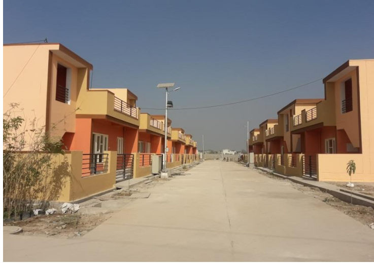
Kota Phase-I in progress.
