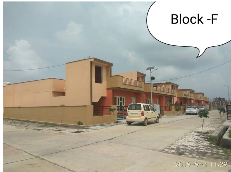
Kota Phase-I in progress.
