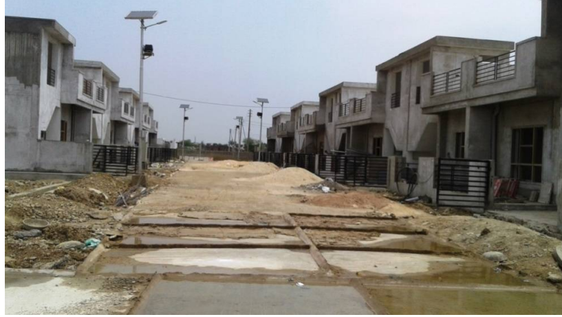
Kota Phase-I in progress.
